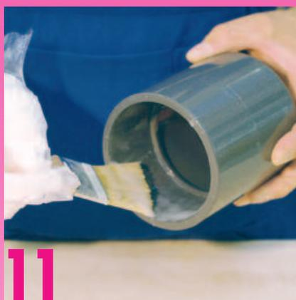
Stir adhesive and soak the brush well with adhesive. Apply a normal layer of adhesive on the inside of the fitting in the direction towards the end of the pipe.
