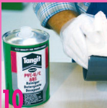
Ensure that both the pipe/fitting are perfectly cleaned. Surfaces to be bonded must be perfectly dry before applying adhesive.
