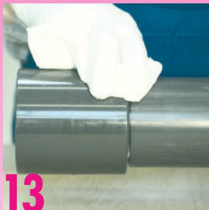
Immediately insert the pipe into the fitting to its full depth without twisting and bring them into the correct alignment. Remove excess adhesive with absorbent paper.
