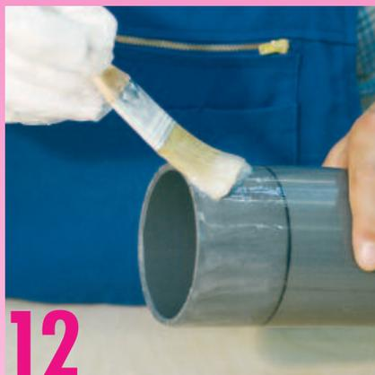
Cover the pipe end axially. Apply a thicker layer to the pipe end with firm brush pressure. The brush strokes should always be in an axial direction.
