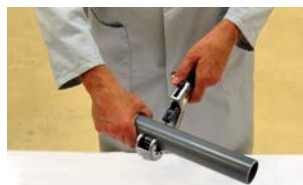
Cutting the pipe to length
