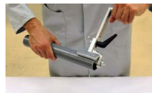
Chamfering the pipe
